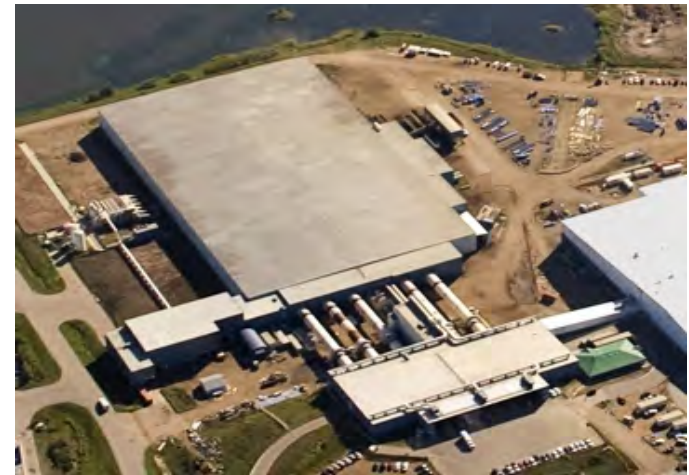
Edmonton Waste Management Centre of Excellence
